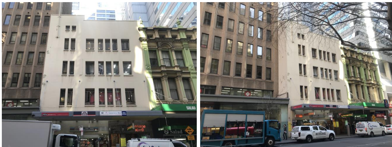
Figure 9 Existing building at 19-21 Hunter Street
