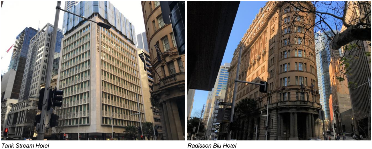
Figure 14 Development to the north of the site
